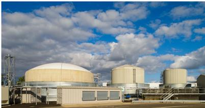
One year after commissioning, the plant is converting 200,000 litres per day of feedstock into renewable energy. This feedstock includes wash waters from the site and 1,200 tonnes of residual bi-products and ingredients per annum.
